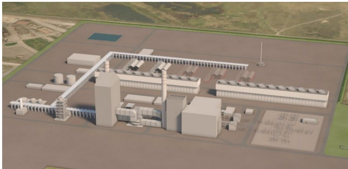
Figure 3: Alternative view of The Net Zero Teesside Project
